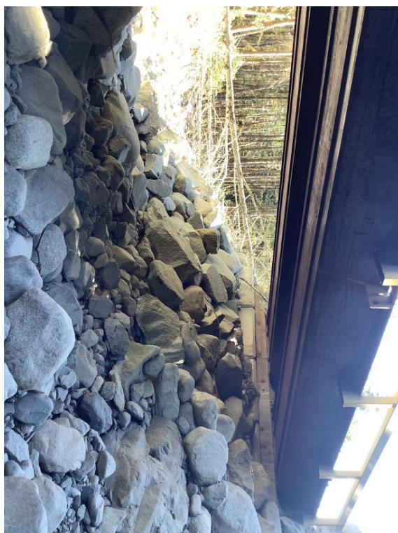
Right Bank Abutment when facing downstream
