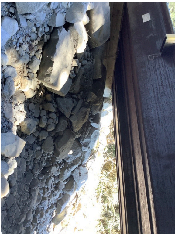
Right Bank Abutment when facing downstream
